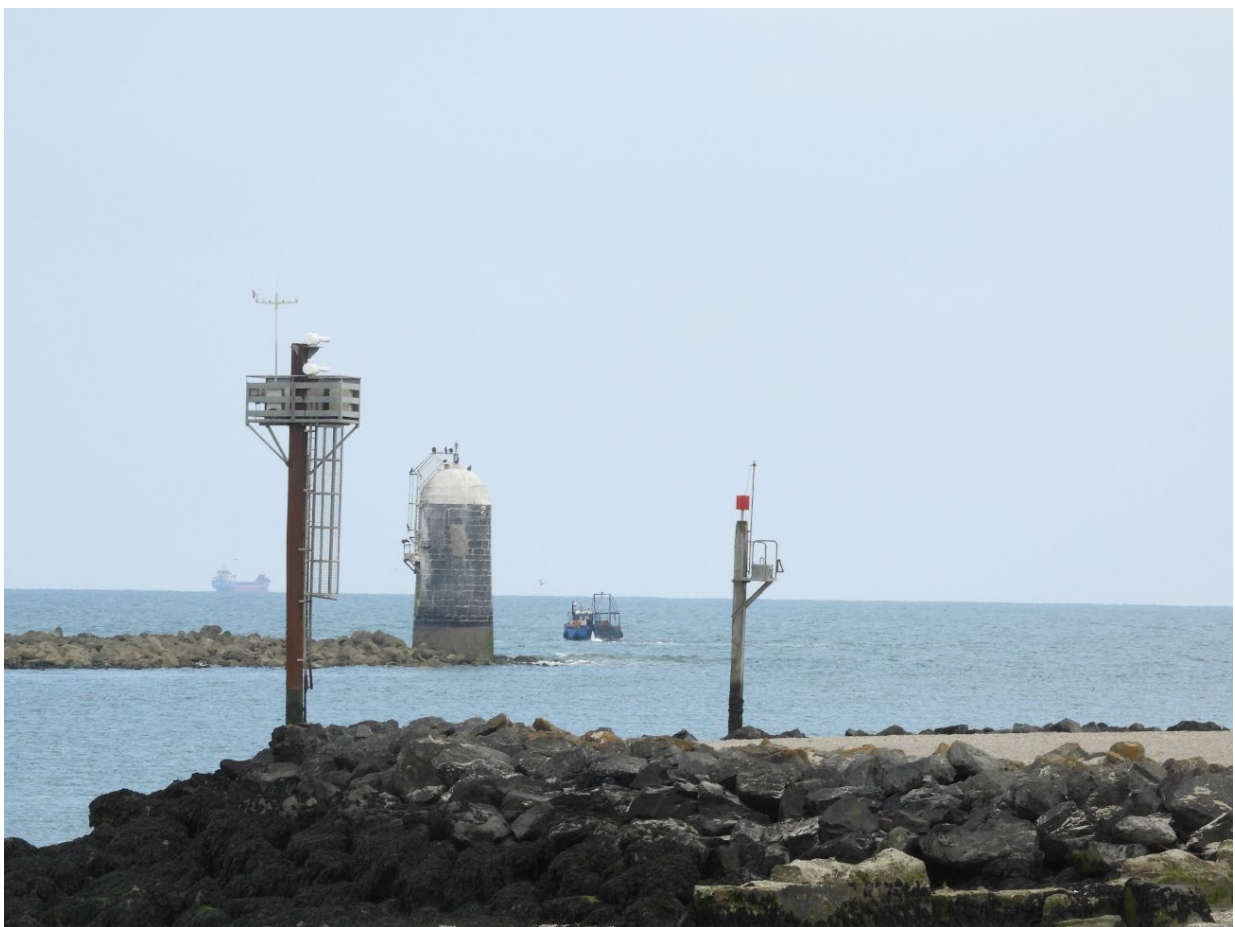
Figure 4 – Image showing a collection of Local AtoN at the entrance to Drogheda Port on the River Boyne, Co. Louth. From left: Port entry Light to delineate the narrow entrance channel, the Aleria Beacon marking the Northern breakwater and a Port Hand Beacon inside the channel
