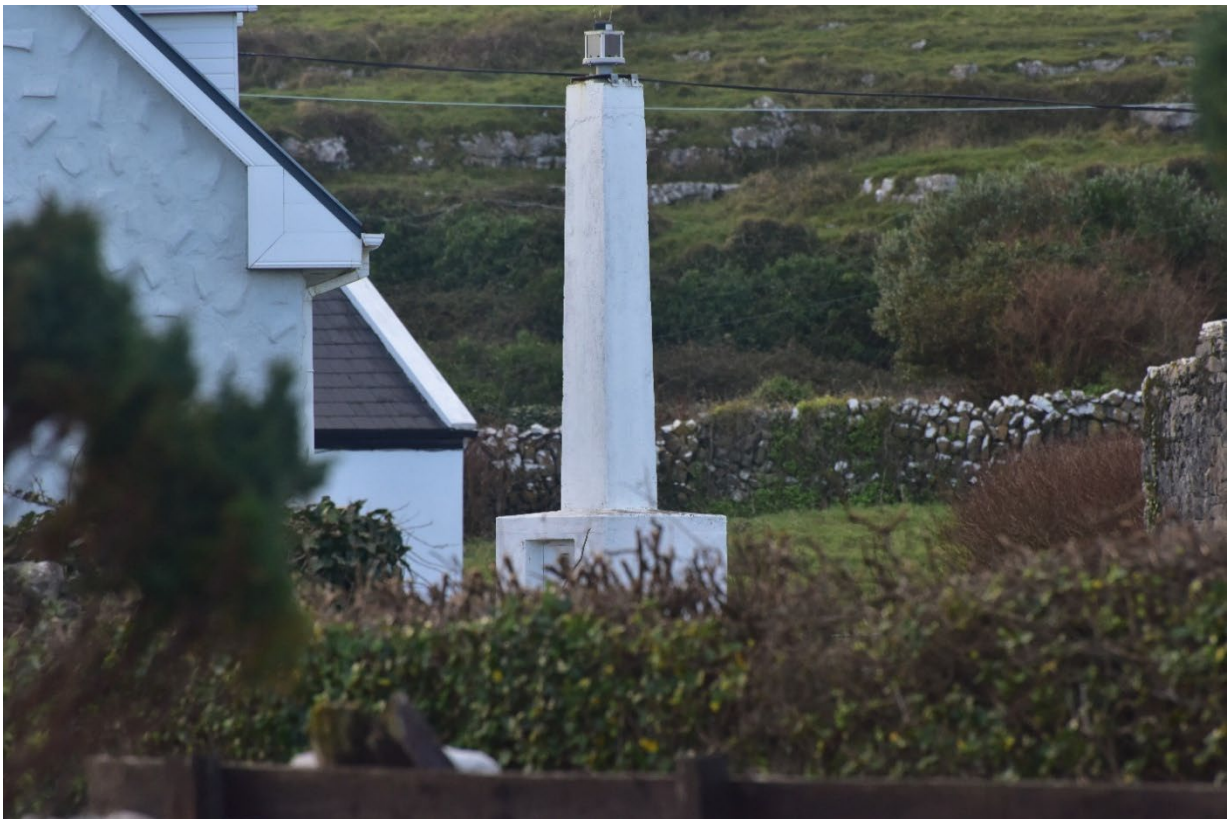
Figure 2 – One of two Occulting White Leading Lights, marking the entrance to Kileany Pier, Kilronan, Inis Mor (Aran Islands)
